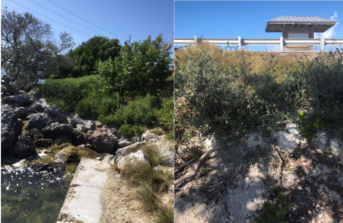
Figure 2-14: Bridge approach near Duck Key, Mile Marker 60.
