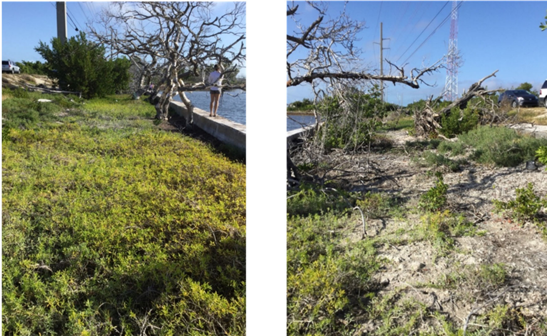
Figure 8-2: West Summerland Key revetment location.
