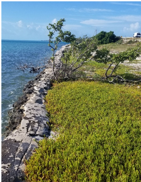
Figure 8-6: Existing sea wall along Indian Key Fill.
