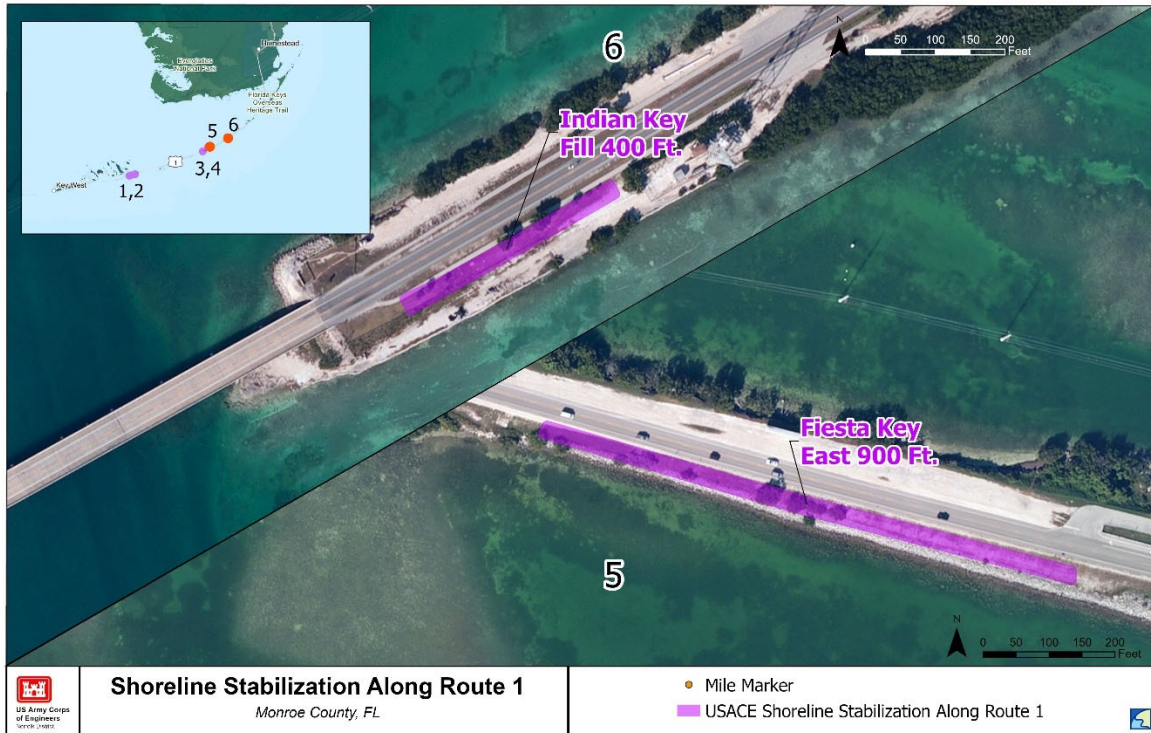
Figure 6-3: Shoreline Stabilization Areas 5 (bottom) and 6 (top)
