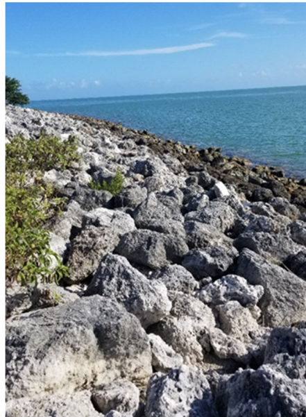
Figure 8-4: Existing rip rap revetment along Fiesta Key East.
