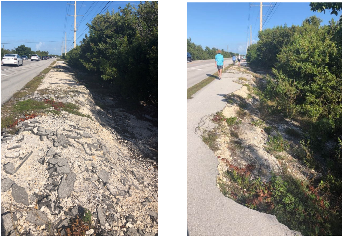
Figure 2-11: Fiesta Key. Near Mile Marker 70 at left, and near Mile Marker 69.5 at right, showing washouts of Overseas Trail.
