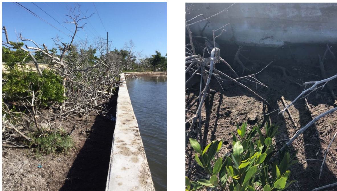
Figure 2-16: West Summerland Key, showing existing concrete seawall and the wetland landward of it. Photo at right shows the base of the wall where water seeps behind the wall.
