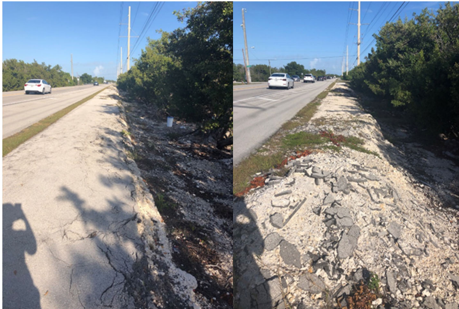
Figure 8-5: Area for the revetment adjacent to the road on Fiesta Key West.
