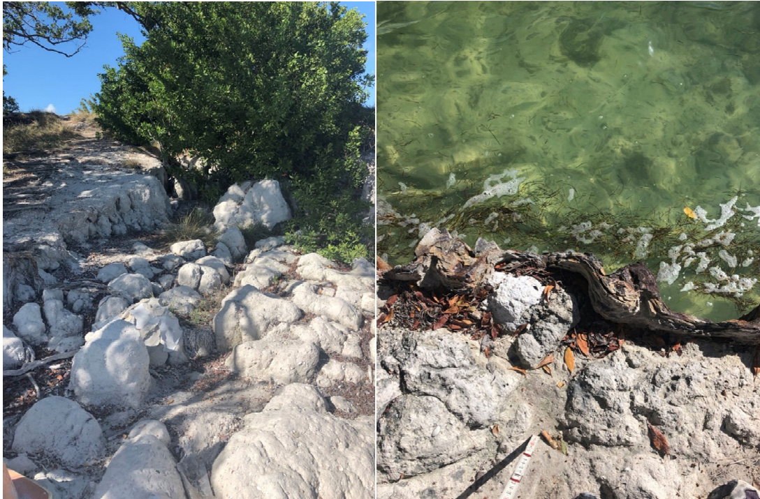
Figure 2-13: Bridge approach near Duck Key, near Mile Marker 61.5
